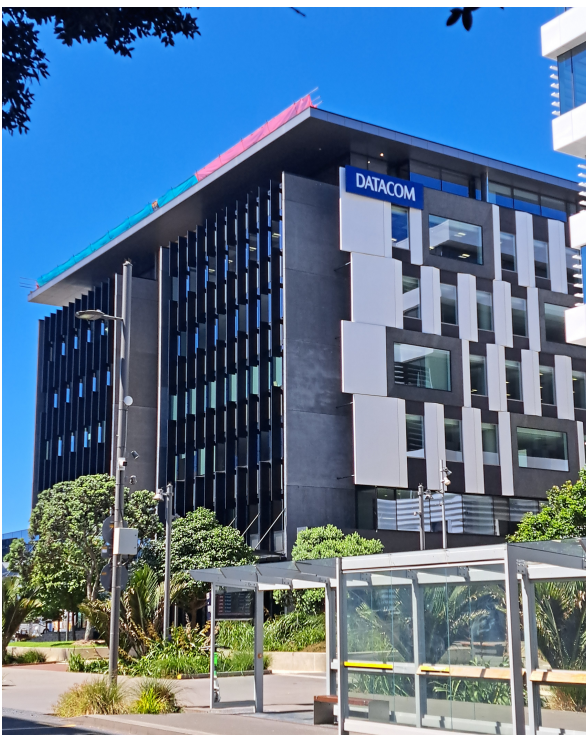
FIGURE 8. Datacom, Auckland, 2025. Courtesy Brian Carpenter.
