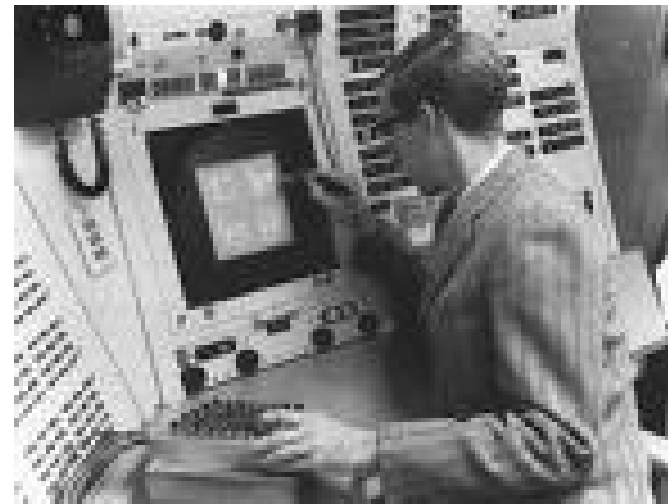
Sketchpad, 1963: Light pen, Constraint-based drawing
